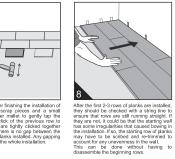
Helpful Hint, After finishing the installation of every row, use scrap pieces and a small harmmer or rubber mallet to gently tap the planks into the click of the previous row to make sure they are tightly clicked together and make sure there is no gap between the long side of the planks installed. Any gapping can compromise the whole installation.
