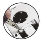
Lubricate the supply pipe ends using a silicone based lubricant and carefully slide the Aquastream™ Thermo unit onto the pipes whilst feeding the low voltage cable through the cable entry point. Secure the unit to the wall using the screws provided (if suitable). Proceed to step 17.
