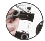
Screw in the two upper fixing screws leaving the heads projecting about 10mm from the wall surface. Feed the working end of the low voltage cable through the entry point in the back plate. Locate the back plate in position on the projecting screw heads. Ease the back plate downwards and engage the screws in the slots. Fix the lower fixing screw and tighten the upper fixing screws.
