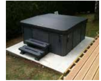
A 10-15 cm concrete base is ideal preparation for a hot tub.
