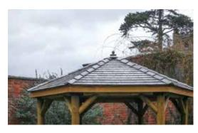
Cedar Shingles used on the roof of Round Timber Gazebos and Forest Retreat Sheds will fade over time to a silvery, grey colour. For maximum life expectancy a suitable cedar cladding oil can be applied.
